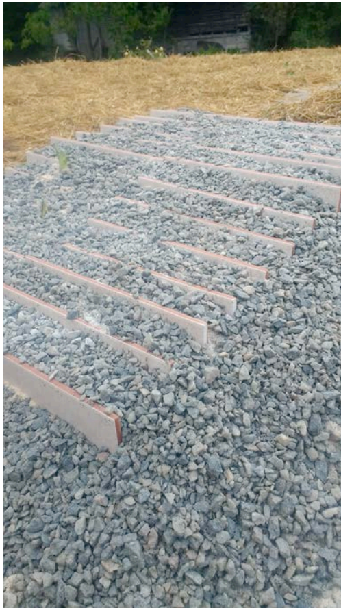
Mix in place, mulched with gravel, and ready for planting
