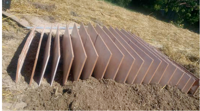
Tiles in place
